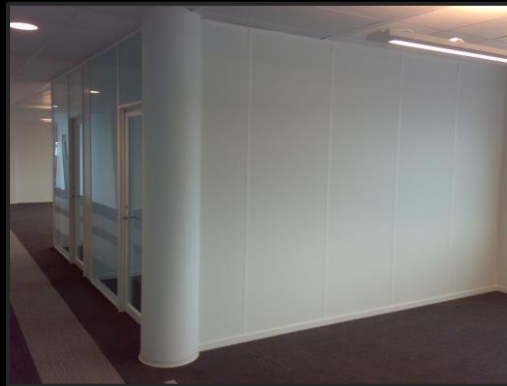
SOLID SYSTEM WALLS V-GROOVE OR U-JOINT
